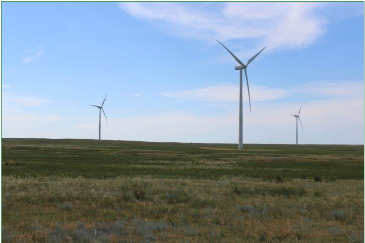
City of Medicine Hat – Box Springs Wind Farm
